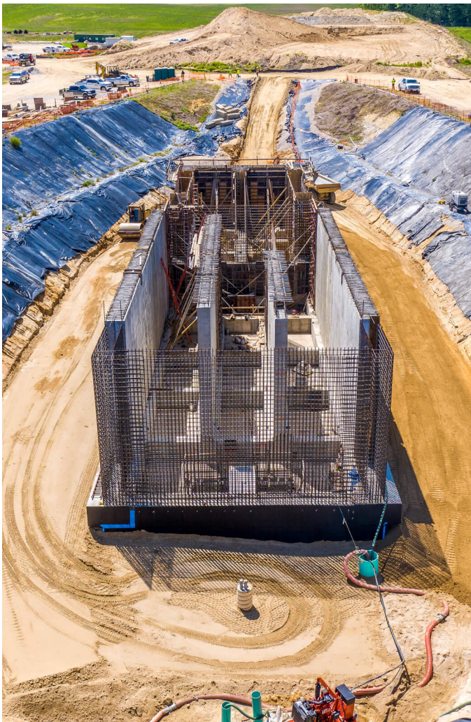
With Sage Intacct, GeoTechnologies Inc. are saving about 15 hours a month in the reporting process.
